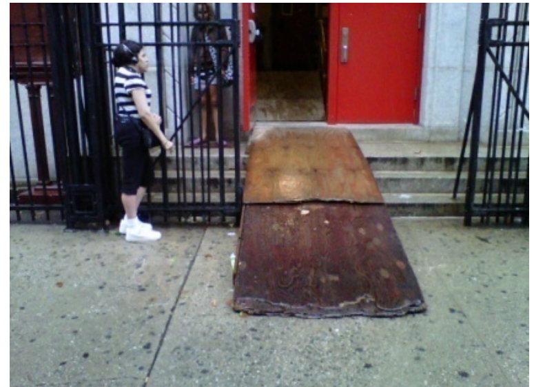
Figure 2: Inaccessible shelter entrance during Hurricane Irene NYC
